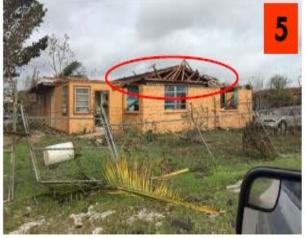
Building Damage Ranking 5: The roof structure is damaged. The right-most portion of the house is missing the roof entirely. Several windows were blown out and the door appears to be missing.
