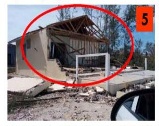
Building Damage Ranking 5: Half of the house is gone, which is classified as wall structure failure and roof structure failure.
