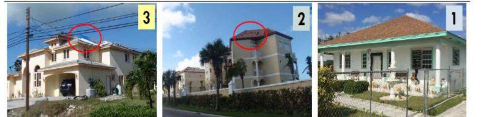
Building Damage Ranking 3: There is major roof cover loss (over 20%) that must be covered to prevent leaks. This is evident by the blue tarp on top. There are no visibly broken windows and doors.
