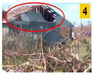
Building Damage Ranking 4: The roof structure is intact, but there is extensive roof sheathing damage. There is no visible window/door breakage. There is partial wall structure failure, but not enough to classify as a 5.
